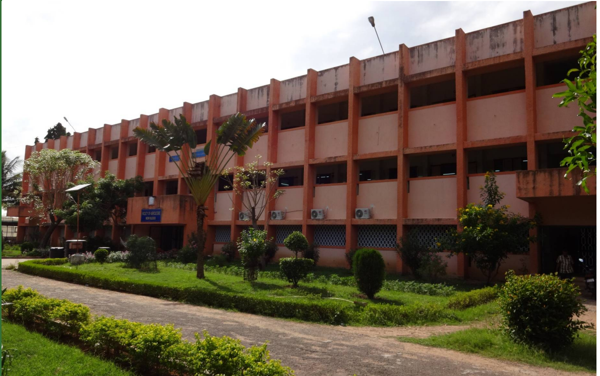
Class Rooms - New Block
