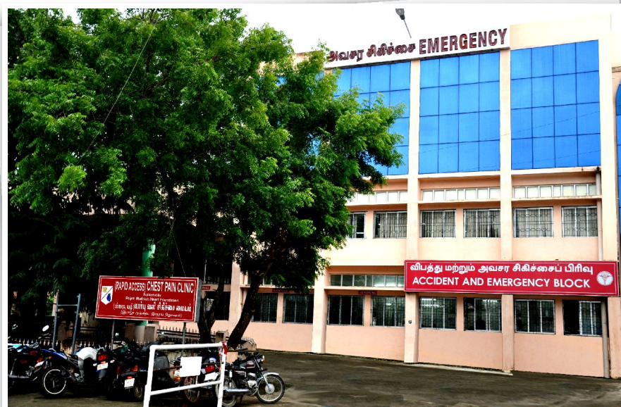
R.M.M.C. HOSPITAL - ACCIDENT AND EMERGENCY BLOCK
